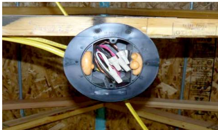
Fix: wide flange box with optional seal vapor barrier to box flange or use foam gasket on the flange. Note: wire openings are sealed with foam.
