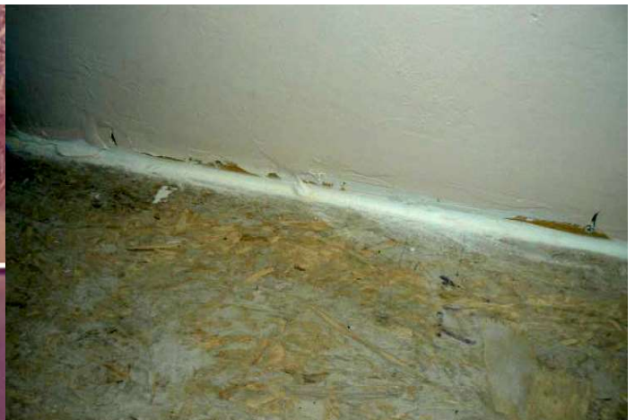
Exterior wall/junction – gap between bottom plate and floor indicates inadequate caulking (left). Fix – seal the wallboard to the floor (right).
