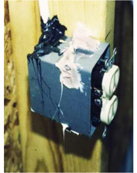
Fix: seal openings in standard box.
