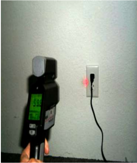
Air leakage at exterior wall electrical outlet.
