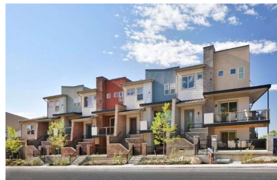
Residential infill development, Louisville, CO (kgarch.com)
