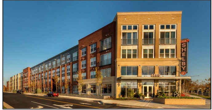
The Shelby in Alexandria, Virginia, wraps 240 dwelling units around 384 parking spaces (KTY Arch. + Planning)
