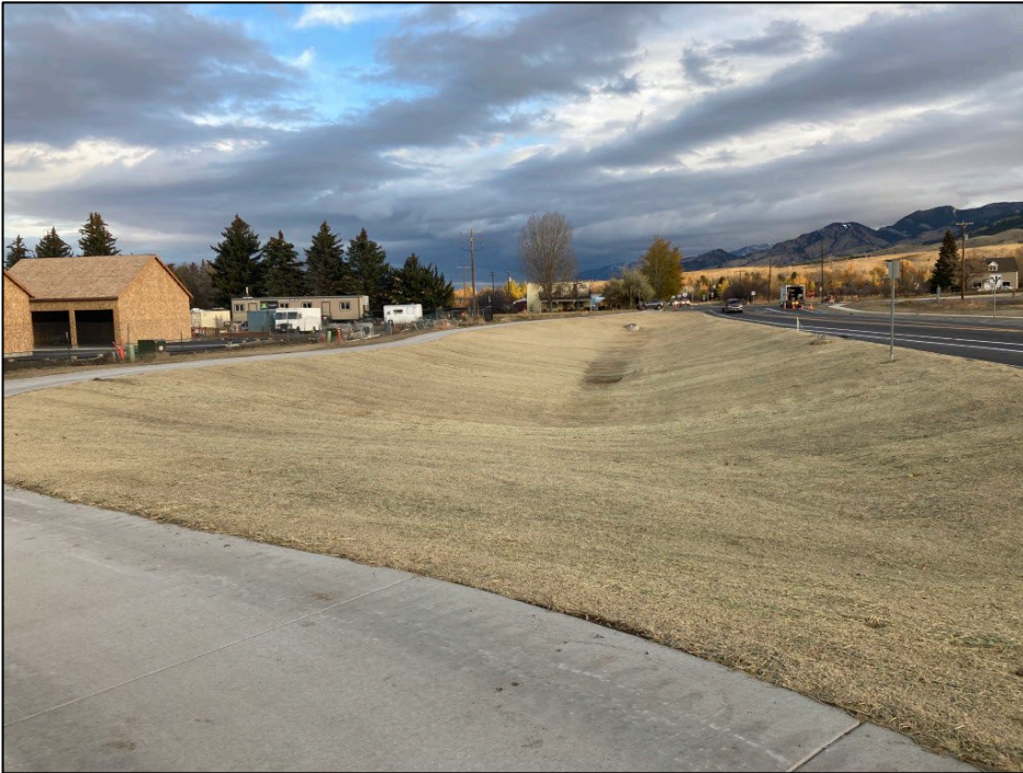
Graphic 5.0.1: Recently constructed and stabilized stormwater pond
