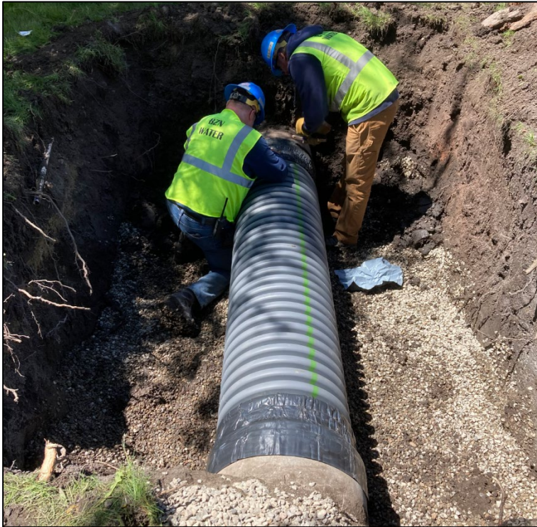
Graphic 2.0.1: Stormwater pipe replacement and repair
