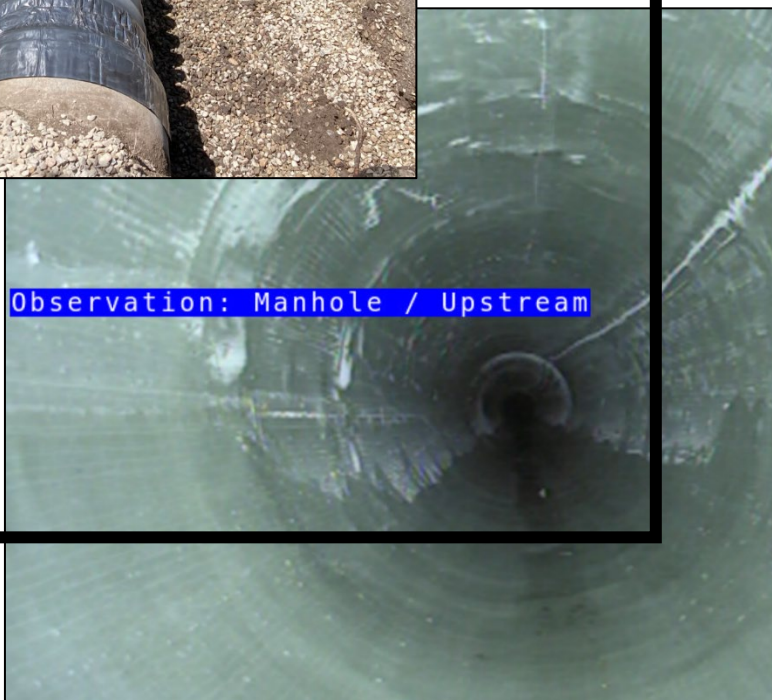
Graphic 2.0.2: Newly installed cure-in-place liner; downtown Bozeman
