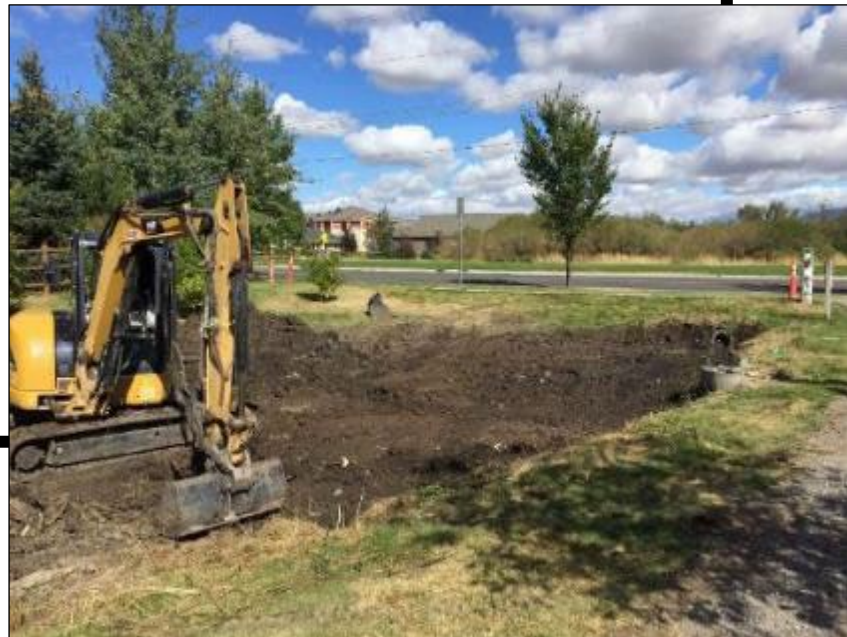
Image 6.0.2 Stormwater basin restoration
