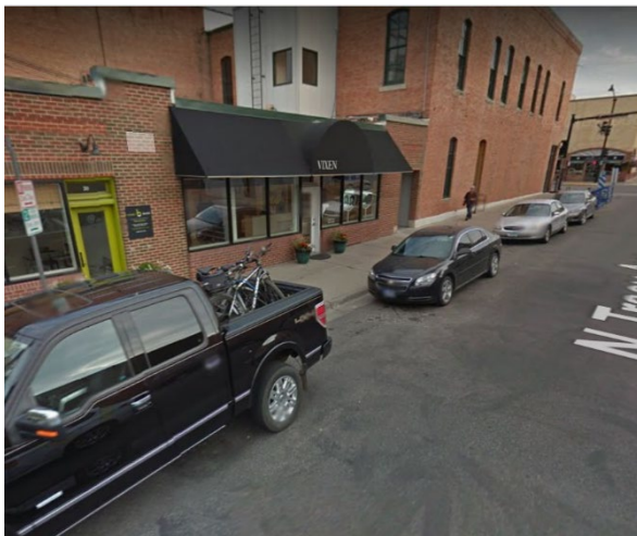
North Tracy Avenue blank wall
