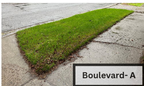
Example of an acceptable before photo.
