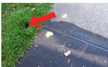
Some leaks result in pressure loss, which may prevent the head from popping up.
