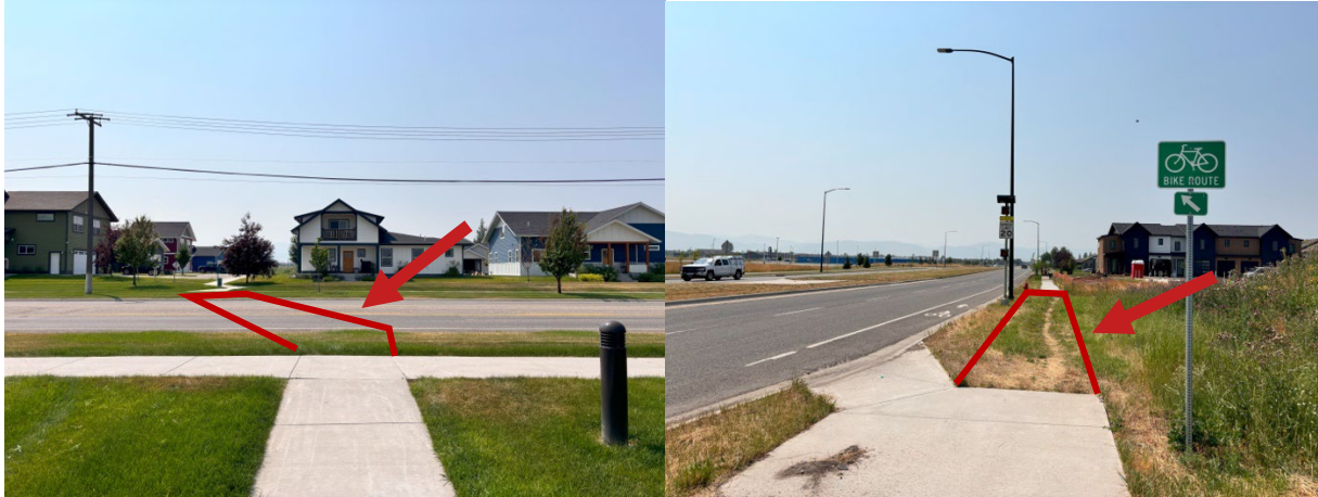
Examples of a “Spot Gap” (left) where neighborhood sidewalk connectors do not include a crossing across Durston Road and a “Linear Gap” (right) where a section of sidewalk is missing along Cottonwood Road
