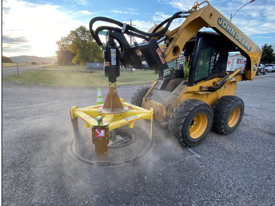
Figure 6 – Example of Mr. Manhole Grade and Casting Repair
