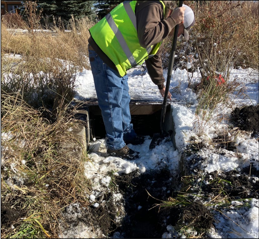
Figure 11 – Curb Chase Cleaning
