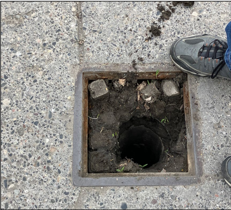
Figure 14 – Undersized Inlet and Lateral on S. Willson Ave. and W. Olive St.
