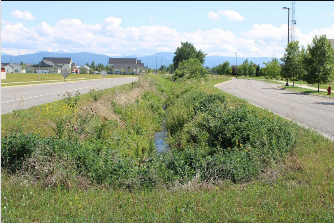
Figure 18 – Vegetation Overgrowth into Open Channel Along Davis Lane
