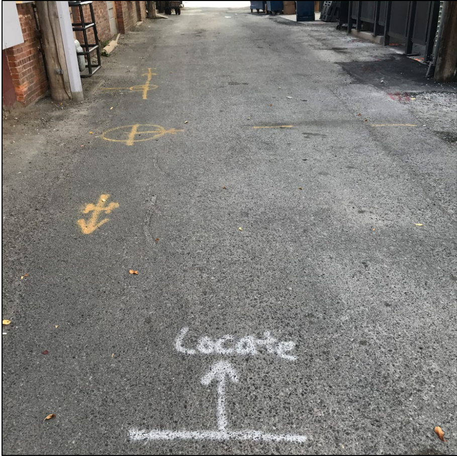
Figure 12 – Utility Locate on Mendenhall St
