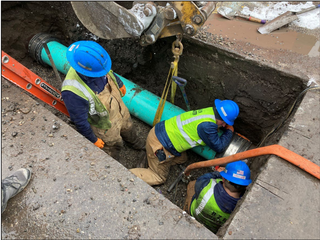
Figure 8 – Storm Drain Repair on N. Church St.
