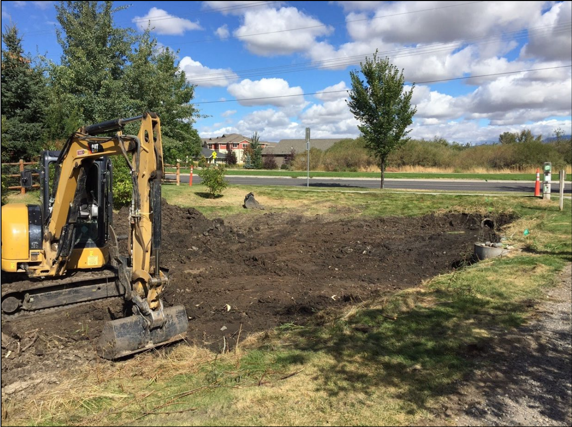
Figure 10 – Sediment Removal Maintenance on a Detention Pond
