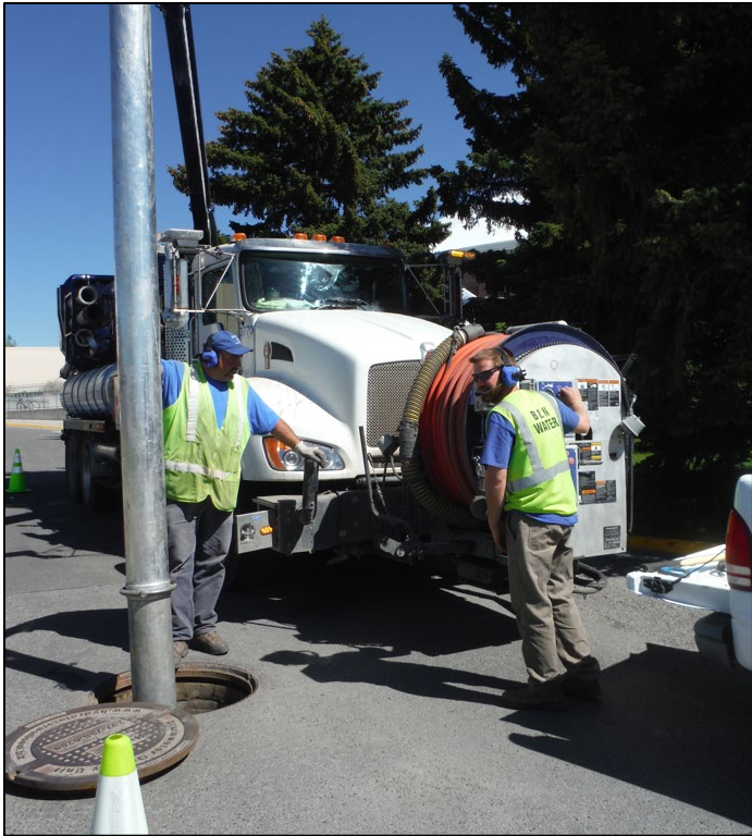
Figure 17 – Vac Truck Cleaning of a Treatment Unit
