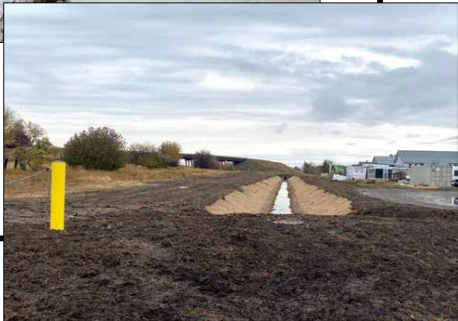
Graphic 2.0.2: Manley Ditch Immediately Following Rehabilitation
