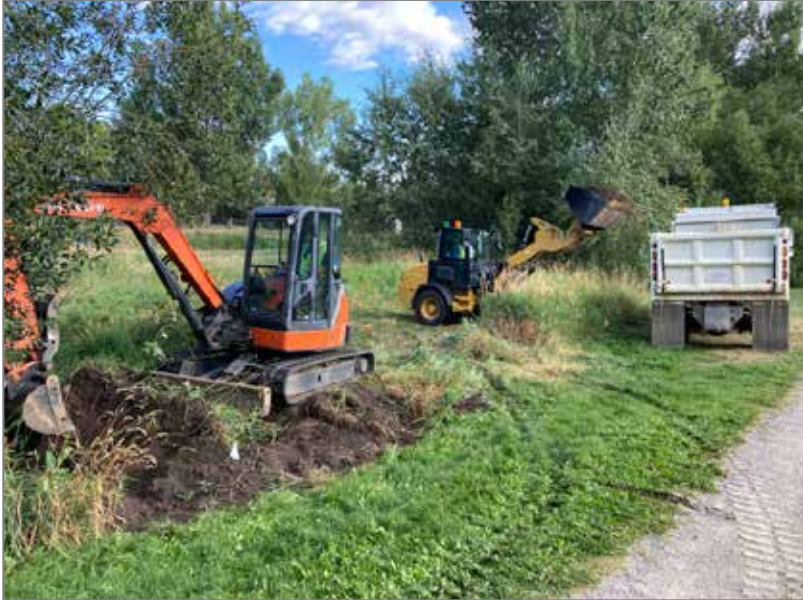
Graphic 6.0.1: Sediment filled post-construction facility during maintenance.
