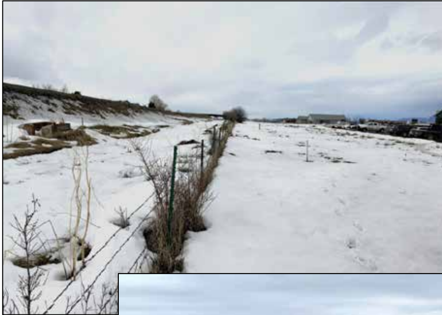
Graphic 2.0.1: Manley Ditch Before Rehabilitation
