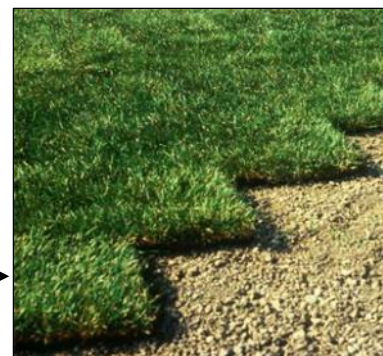
Stabilize Disturbed Area Sod →
