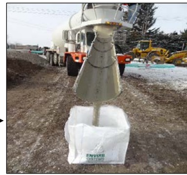
Control Concrete Waste Washout Bag →
