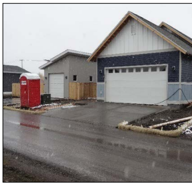
← Contain Disturbed Area Straw Wattle
