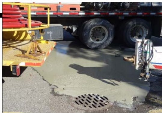
Image 4 - Construction-related pollution event
