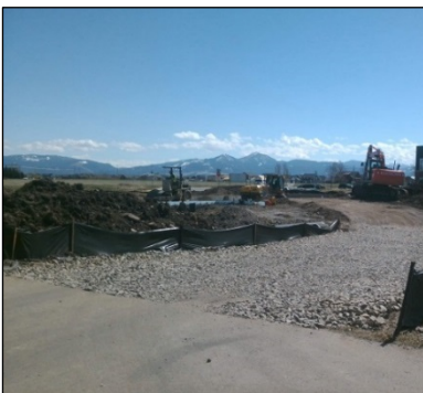
← Mitigate Tracking Gravel Drive Entrance
