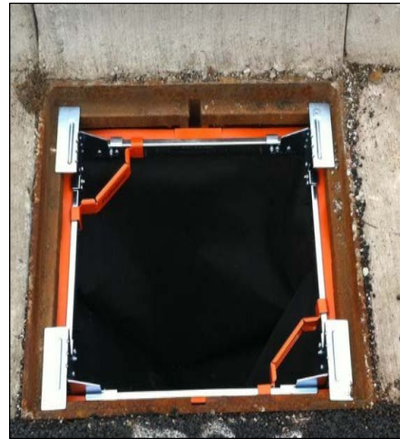
Image 21 - Installed inlet protection. Image taken from www.ADS-Pipe.com
