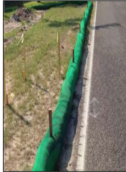
Image 13 - Properly installed filter sock. Image from filtrex.com
