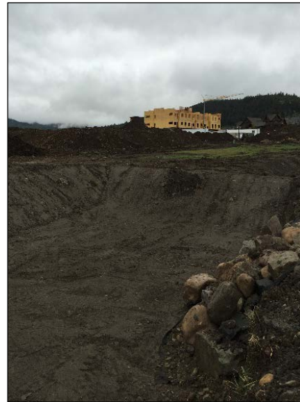
Image 20 - Sediment trap and armored overflow
