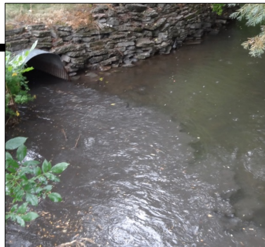
Image 2 - Stormwater dumping into Bozeman Creek
