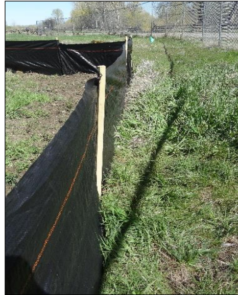
Image 18 - Properly installed silt fence
