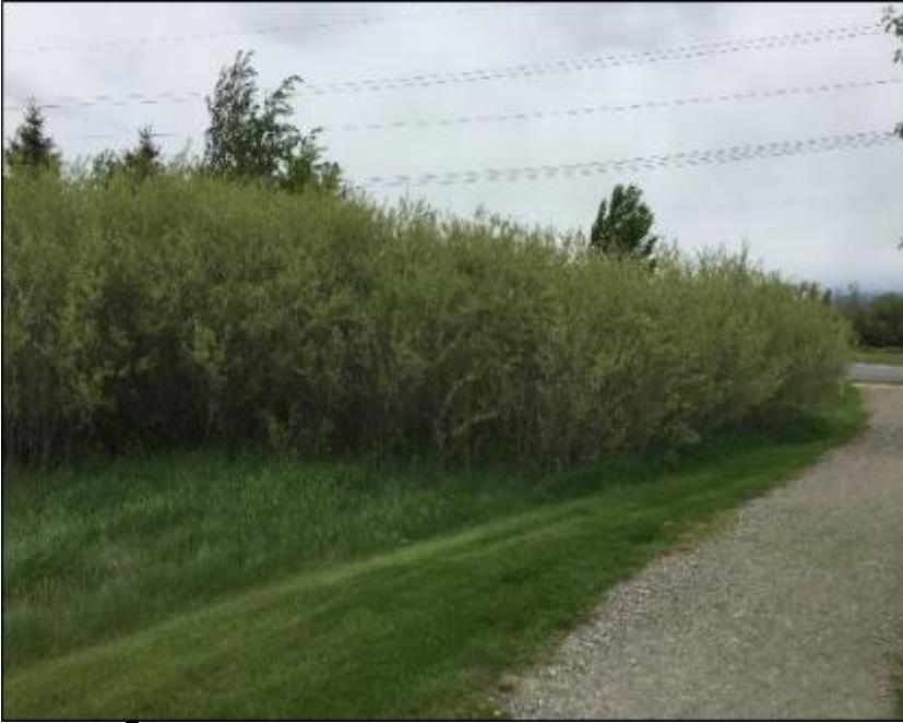
Image 6.0.1: Overgrown stormwater basin
