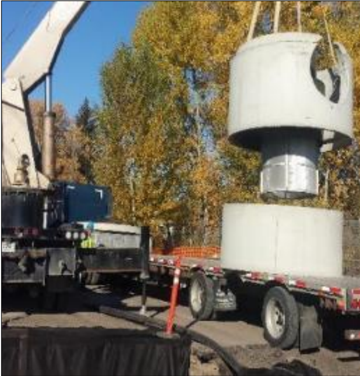
Image 2.0.1: Stormwater treatment unit installation
