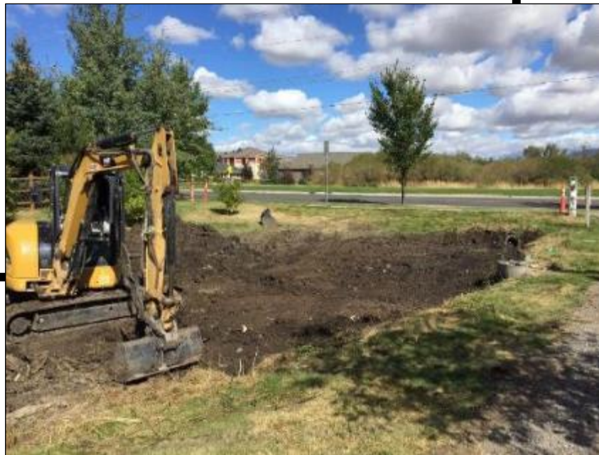
Image 6.0.1: Dredged stormwater basin
