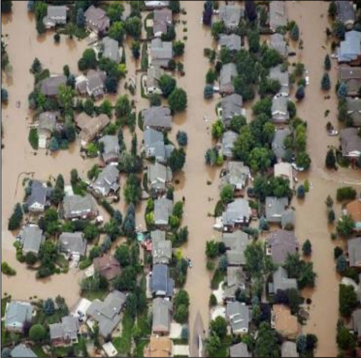
Image 1.0.1: 2013 Colorado urban flooding. Source: theatlantic.com
