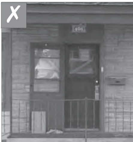
If a door requires replacement keep the original door proportions.
