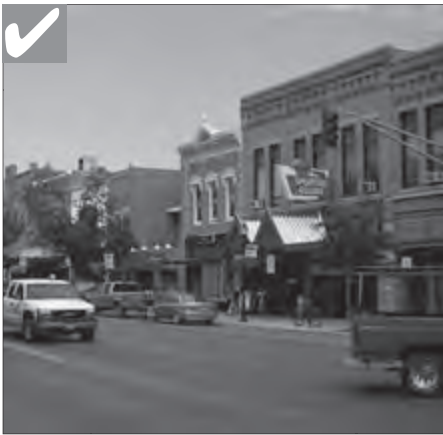
A strong alignment of horizontal elements exists along the street, this quality should be maintained.
