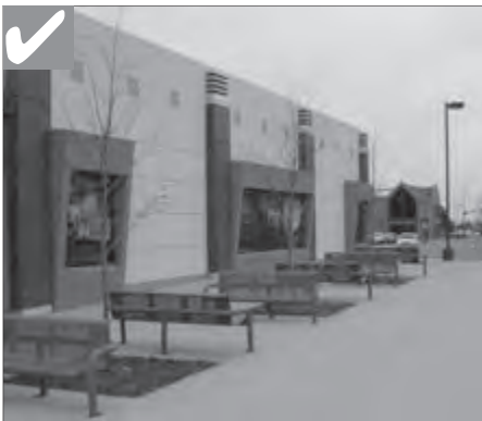
A successful method in creating an attractive street edge includes providing display cases.
