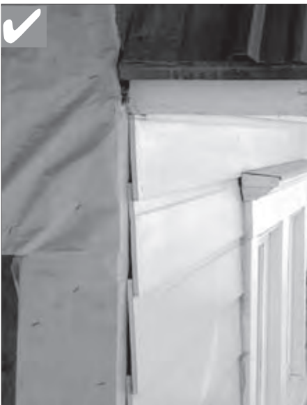
The use of hardiplank horizontal lap siding is appropriate in most residential neighborhoods outside of the historic district.
