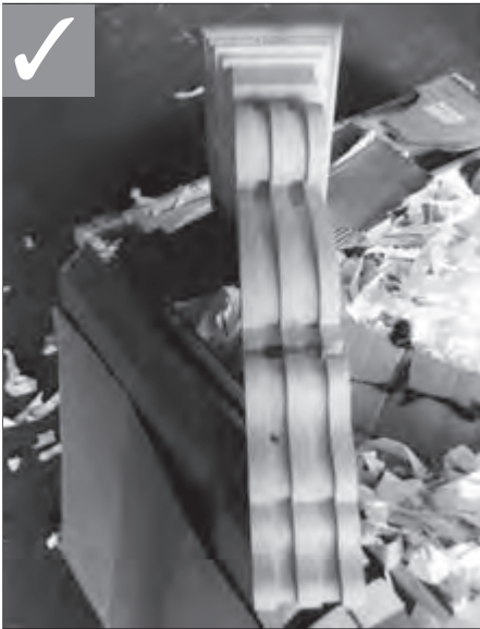
When reconstruction of an element is impossible, develop a new design that is a simplified interpretation of it.
