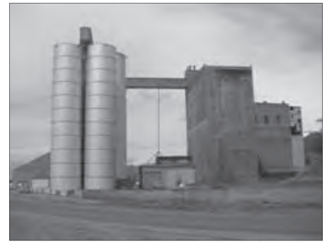
The Historic Story Mill complex uses many different materials such as wood, metal, and stone.
