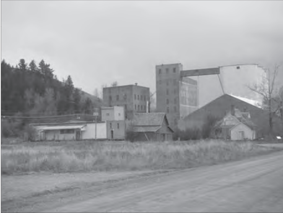
Story Mill Historic District
