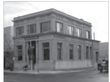
The National Bank of Gallatin Valley (1 W. Main) exhibits another unusual material-concrete blocks molded in imitation of rusticated masonry.
