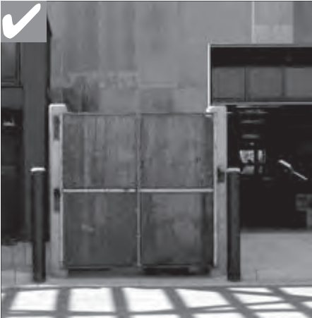
Service areas should be visually unobtrusive and should be integrated with the design of the site and the building.
