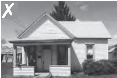
The porch on the left has experienced an inappropriate alteration; enclosed railing. Compare it with its “rehab” in the photo to the right.
