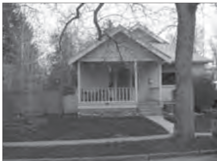
Front porches address the street.
