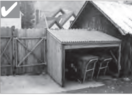
Minimal shed structures, such as this may be utilized at the alley edge.
