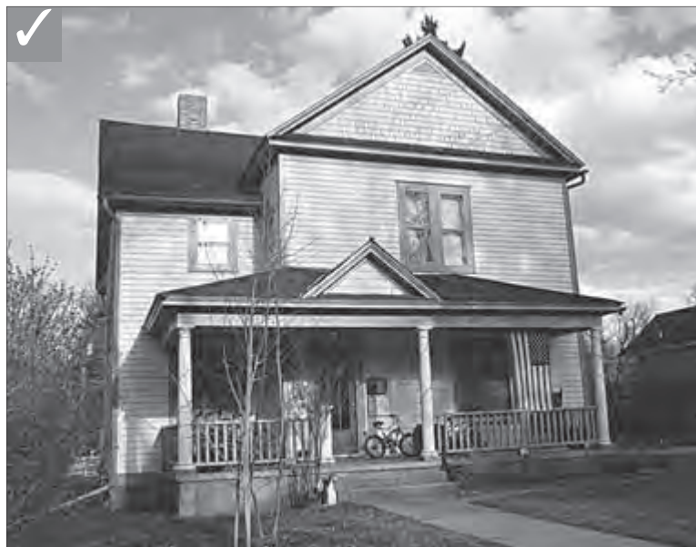
Consider removing later covering materials that have not achieved historic significance. Compare the left photo with the photo on the right, after the synthetic siding was removed. Note how the lap dimensions on the original siding are much smaller.
