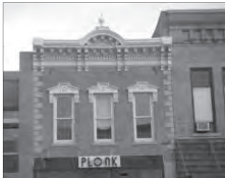
Italianate Commercial Building - upper facade.
