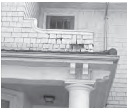
Do not remove damaged materials that can be repaired. In this case, loose shingles may be re-secured while missing ones may be replaced.
