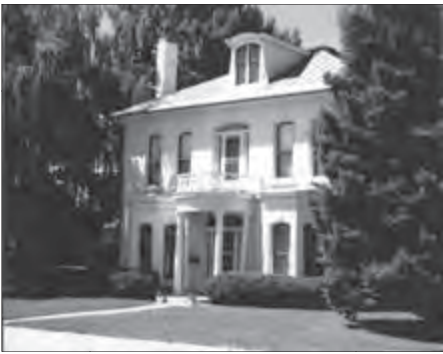
Colonial Revival (Courtesy of the Gallatin Historic Society)
