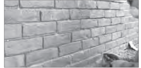
Commence with building cleaning after any repointing has completely cured.
