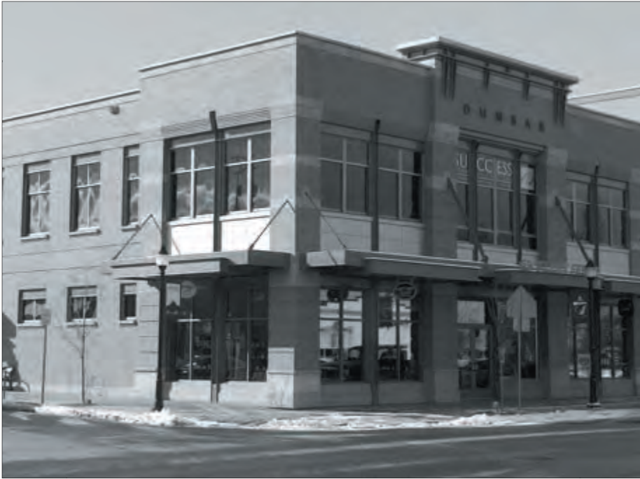
Appropriate new infill building for the commercial character area.
